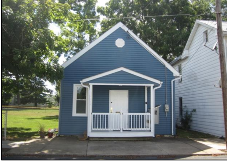
Former AME. Zion Church Building, 211 North Arch Street, Mechanicsburg
